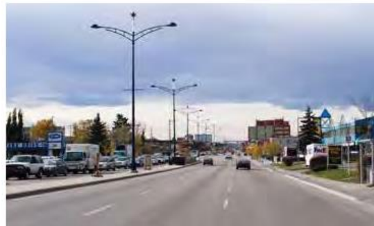
Photo: 16 Avenue N
