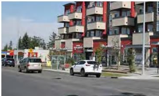
Photo: Centre Street N
